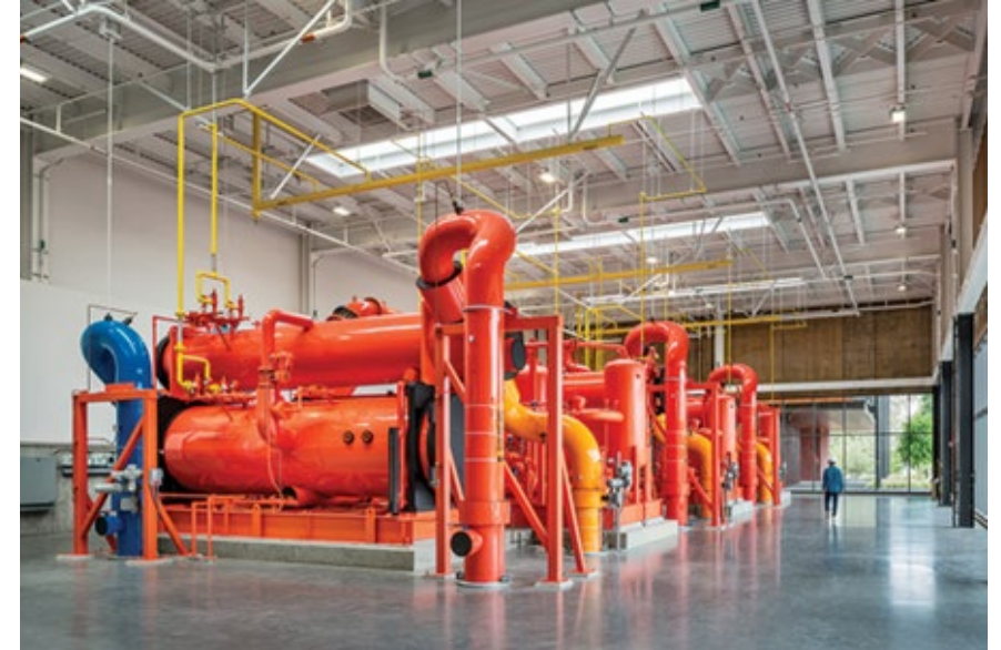
Heat recovery chillers at Stanford
