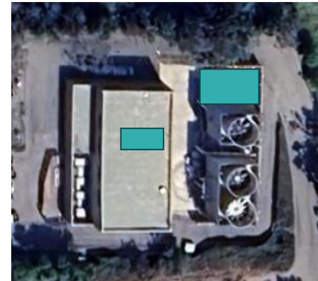
New chiller, cooling tower and pumps
